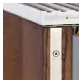
Top of door; exterior view.
